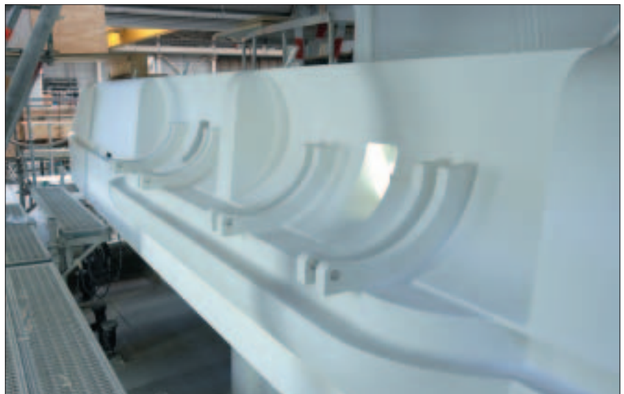
This complex section of the upper-deck bulwarks houses two life-raft canisters. Fair and true surfaces with straight facets and diligently ground welds will require less fairing, which translates to reduced weight and labor costs.
